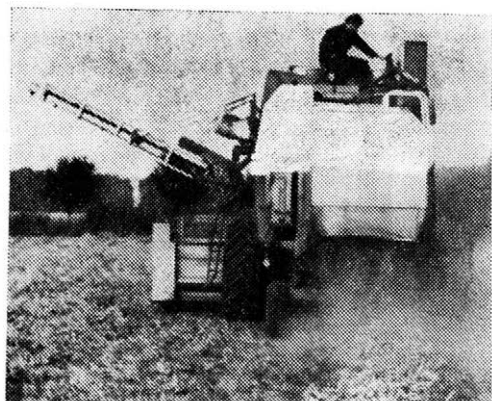
3. Modelová úprava E-512 (1983) pri zbere a výmlate hrachu na pozemkoch JZD Kunovice — Model adaptation of the E-512 combine (1983): harvesting and threshing peas in the fields of the Kunovice co-operative farm
